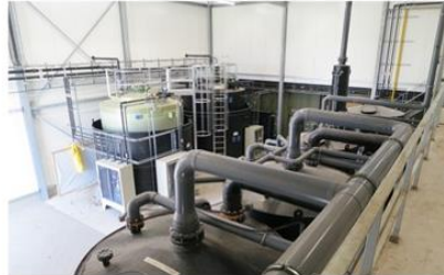
Storage of liquids
